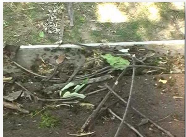
**A gutter guard that sits flat will trap debris. This debris can cause water to flow over the system or flow backwards towards the roofline.**
