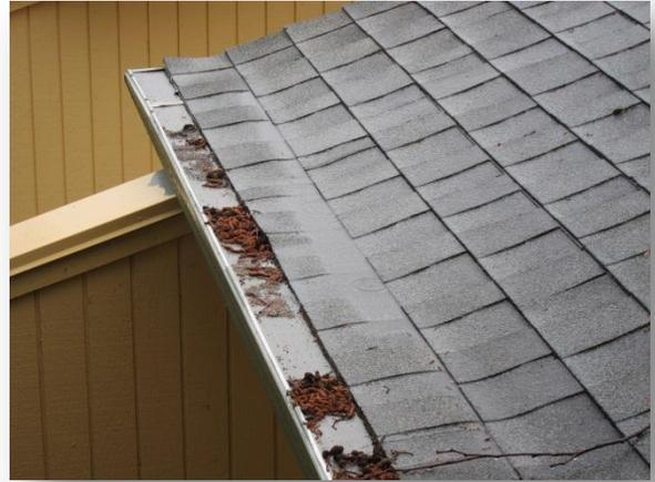
**This system is not just trapping debris, it's causing water to pool on the shingles, behind the gutter guard.**
